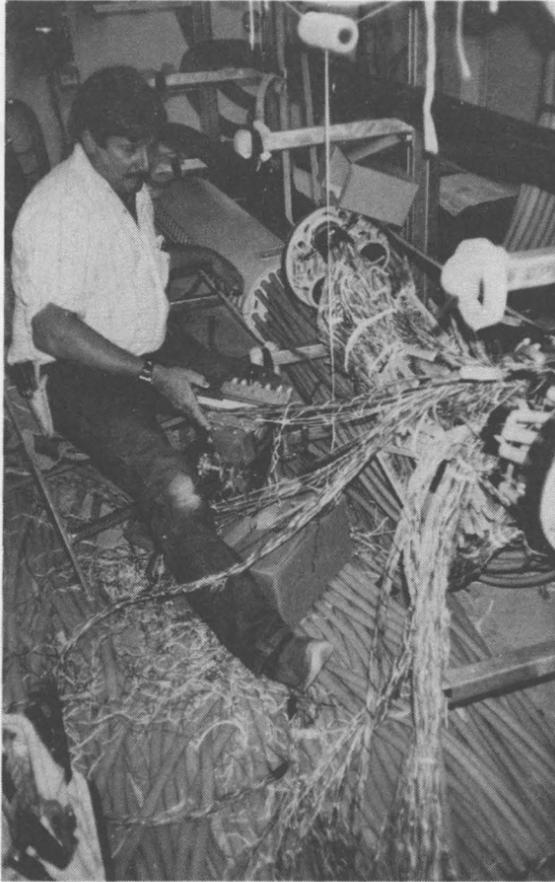
**MICHAEL CROCKER, a US West employee, splices wires that will enable the Sandia telephone switch to connect its customers. The sight of 4,200 pairs of tiny wires might be overwhelming for most, but Crocker knows exactly where to connect every wire.**
