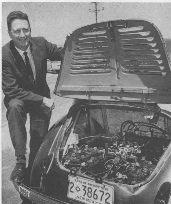
PAUL STICKLER (now retired) in 1963 photo above showed the "Little Joule's" power plant soon after he converted the car into an electric vehicle. It could go 17 miles and up to 40 mph. In photo at right, he shows the electric motor and controller he used in the "Little Joule" and that he keeps today.
