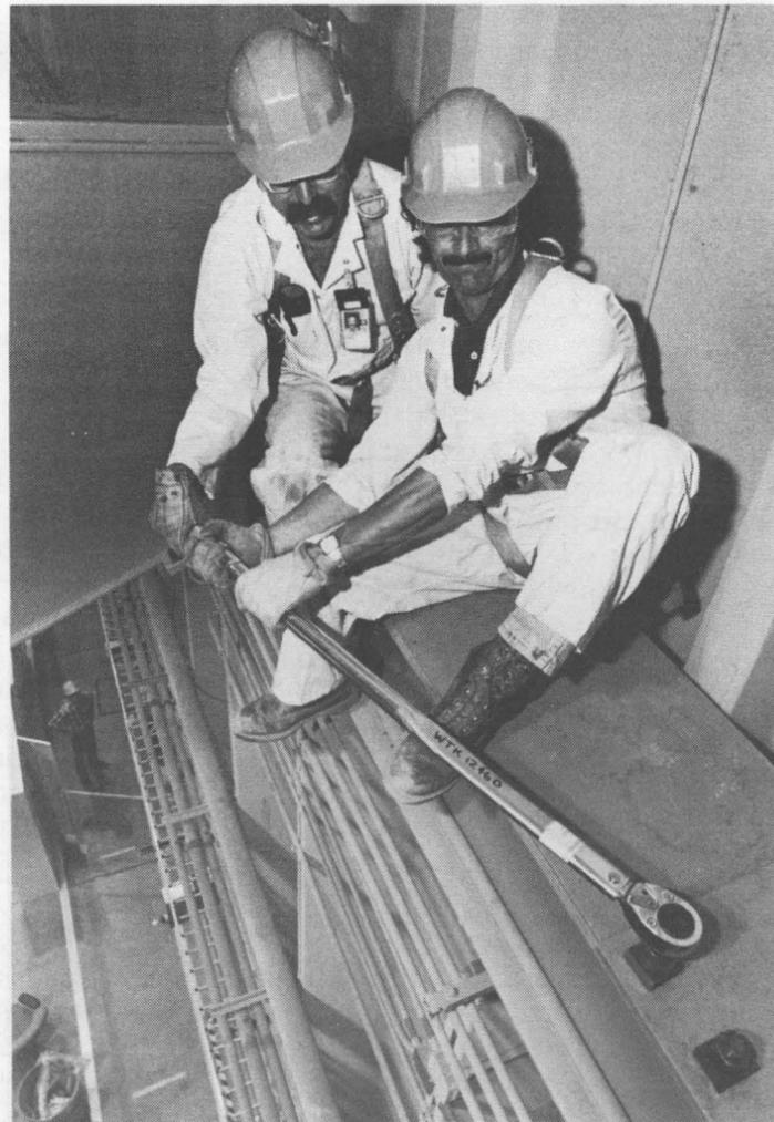
PRECARIOUS PERCH 30 feet above the floor — Sandia tradesmen Richard Parker (7814, left) and Mike Pacheco (7813) are harnessed to a high-bay bridge crane in Bldg. 820 as they tighten a fastener using a torque wrench. Richard and Mike are two members of the Operation Crane Rescue Project that worked on critically needed cranes and hoists during the last holiday break. Reggie Tibbetts, Supervisor of Crane, Hoist, and Rigging Team 7813-3, watches from below.
