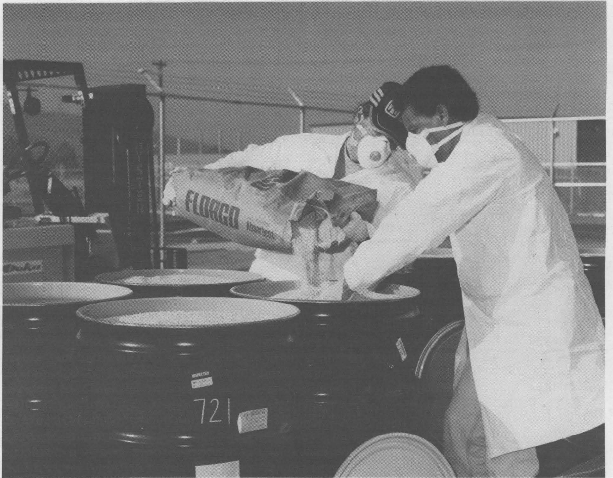
PACKING IT AWAY — Contractors Gus Martin (left) and Jerry Parker pour absorbent packing material into drums being prepared for shipment. They have been clearing out Sandia's Tritium Research Laboratory, making it into a nonnuclear, low-hazard facility.
