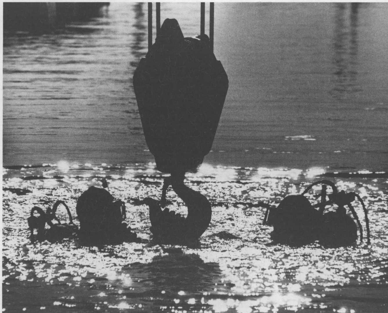
WET WORK — Divers orient a crane hook that removes test equipment from the pool.
