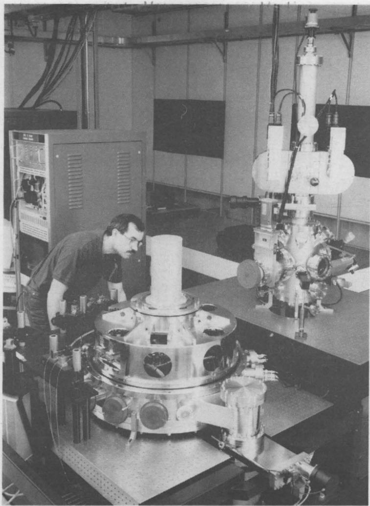
**FINE ETCHING** — Yon Perras (8414) assembled most of the components of the extreme ultraviolet advanced lithography tool, which he is inspecting here at Sandia/California's Advanced Lithography Facility.
