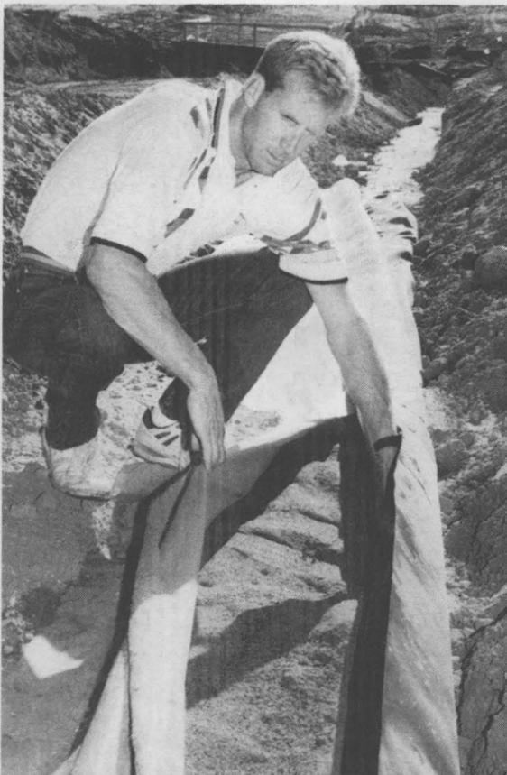
**CHECKING IT OUT** — Steve Dwyer (6621), project manager for the Alternative Landfill Cover Demonstration project, checks out the synthetic liner and sand strata that make up two of the layers of a landfill cover. The project is designed to test a number of cover designs optimized for performance in arid environments.
