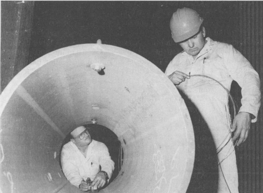
IN PREPARATION for cargo hold tests, Jeff Bobbe (left) and Mike Arvisó (both 6642) install thermocouples on Sandia's simulated nuclear material transport cask, a five-ft-long, two-ft-diameter steel pipe. (Photo by Diana Helgesen, 2732)
