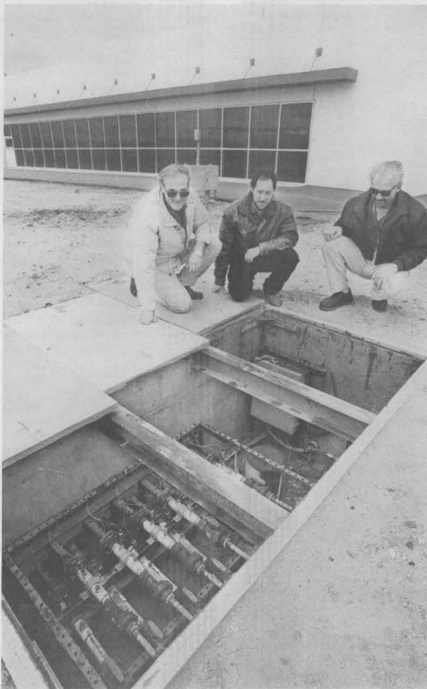
**UNDERGROUND EXPERIMENTATION** — From left, Bill Sullivan of Geothermal Research Dept. 6111, Rico Ortiz of Architecture and Engineering Dept. 7832, and Michael Quintana of Photovoltaics System Components Dept. 6219 examine the instrumented piping leading to underground heat exchangers, part of an experimental renewable energy system that helps heat and cool Bldg. 848 (background).
