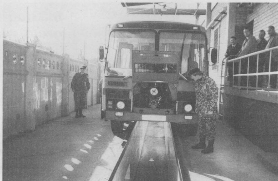
AMONG the physical security improvements at the Ignalina nuclear power plant in Lithuania is this inspection trench similar to a 10-minute oil change bay. From this pit, guards can inspect the undercarriages of vehicles entering or leaving the plant.
