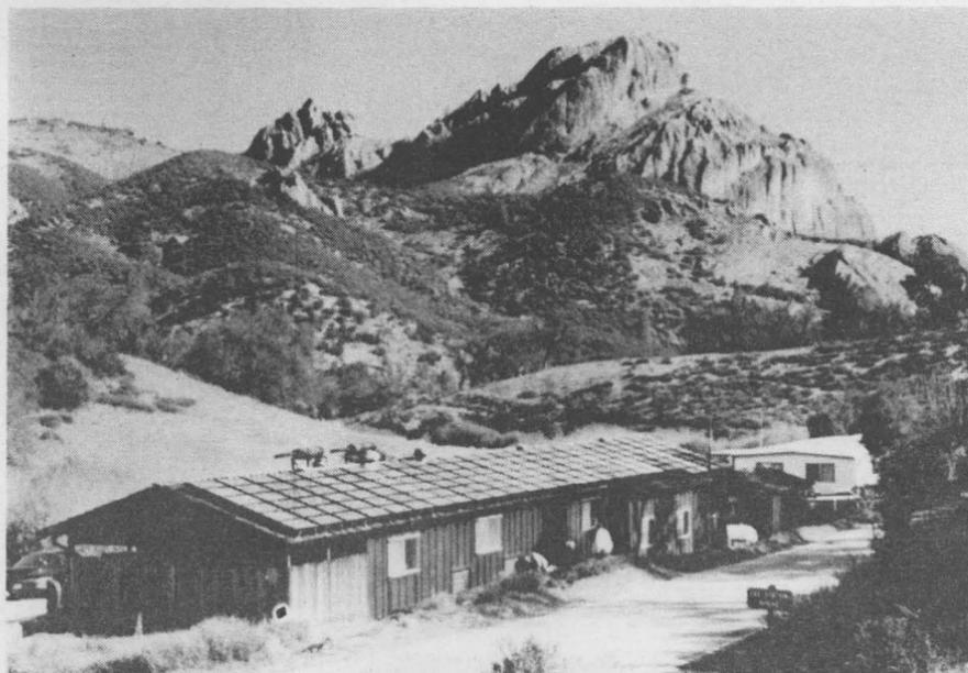
**PINNACLE OF POWER** — State-of-the-art photovoltaic system at Pinnacles National Monument, Calif. The photovoltaic system, including the array on the building's roof, replaces two aging diesel-powered generators and provides power to the service facility at Chaparral, on the west side of the park. The facility includes three ranger residences, a ranger station, visitor center, maintenance workshop, and campground.
