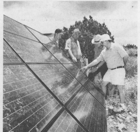
Inspecting the photovoltaic array at Salinas are, from left, Mike Schneegas, National Park Service; Mike Thomas (6218); Glenn Fulfer, National Park Service; and Hal Post (6218). The 24 Solarex MSX-60 modules provide an aggregate output of 1,440 watts.
