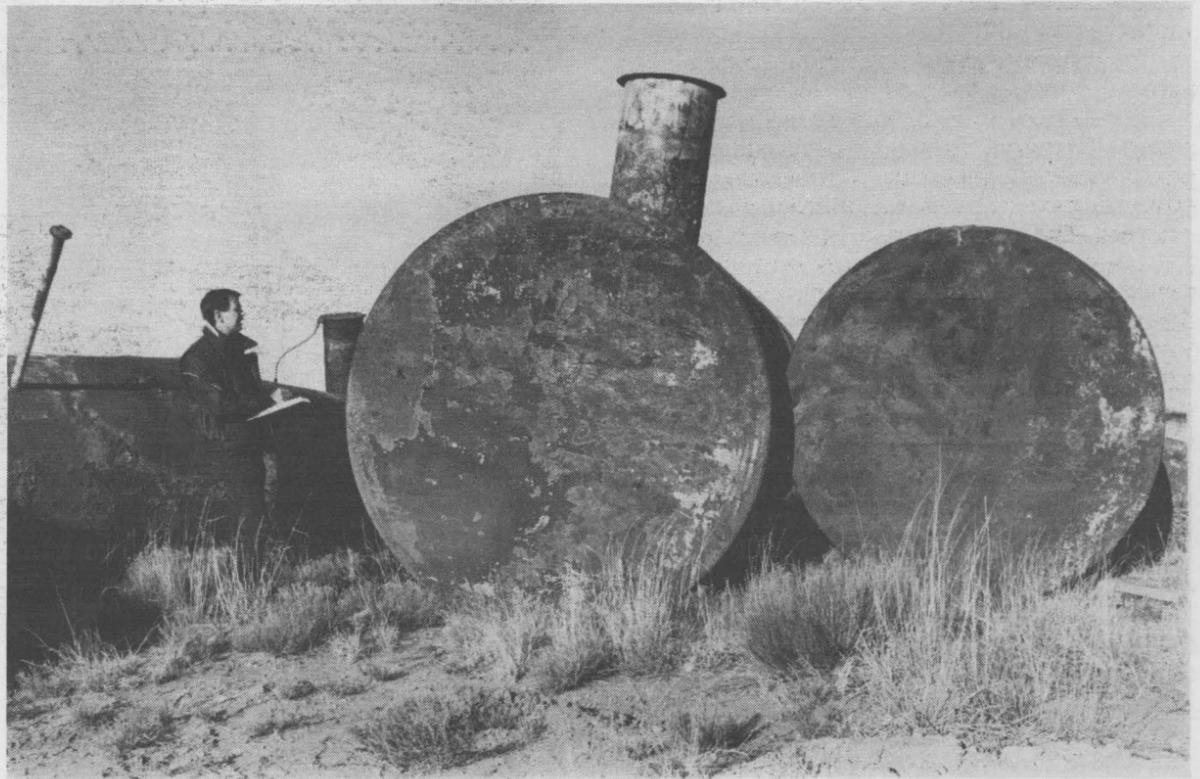
**TRACKING TANKS** — In this 1989 photo, Sandian Dave Dionne checks the condition of underground storage tanks removed in late 1988. According to state and federal requirements, all USTs must be accounted for, brought into compliance with new regulations, closed in place, or removed by December 1998. (Photo by Randy Montoya)
