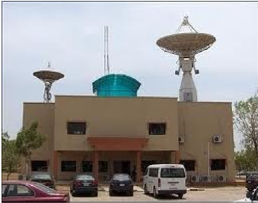
Nigerian Earth imaging satellite control center
