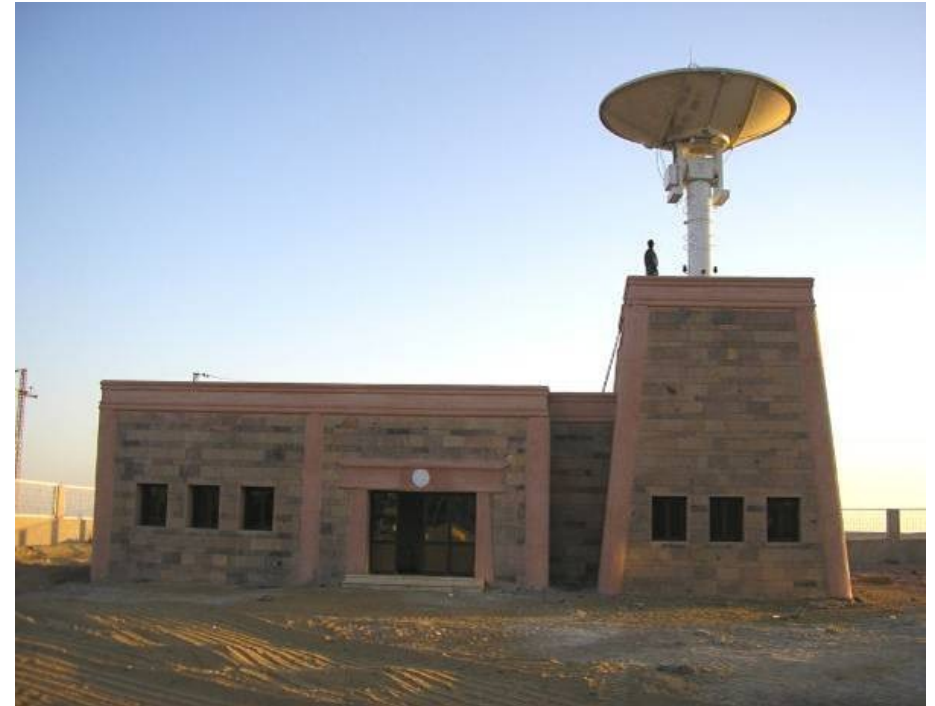
Control center at Aswan
